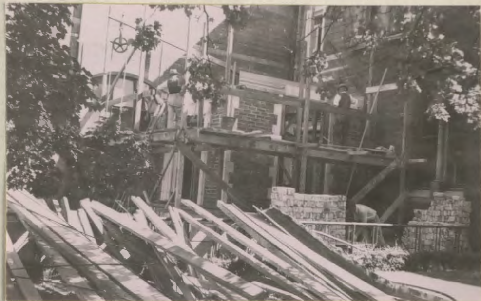
ALTERATIONS IN PROGRESS 1950.
