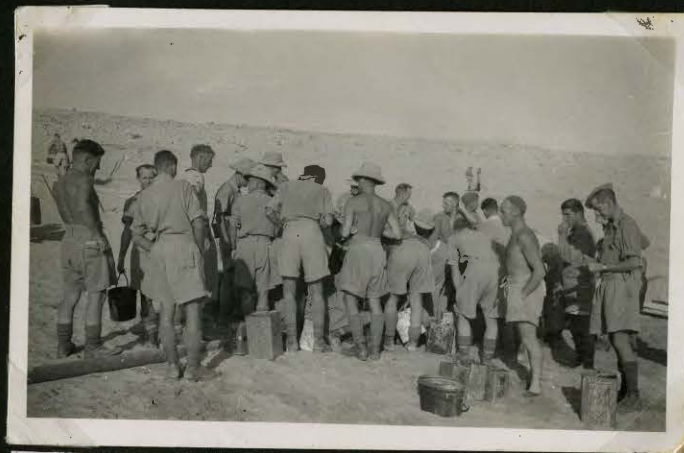
Getting water from a leak in the water pipeline, laid by Engineers to "Kaponga Box" area in July. Very hot. I couldn't spit. I'm in middle, with topee & back to camera.
