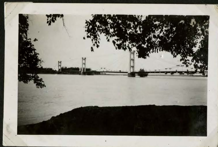
Bridge over Euphrates at Deir-ez-Zor.
