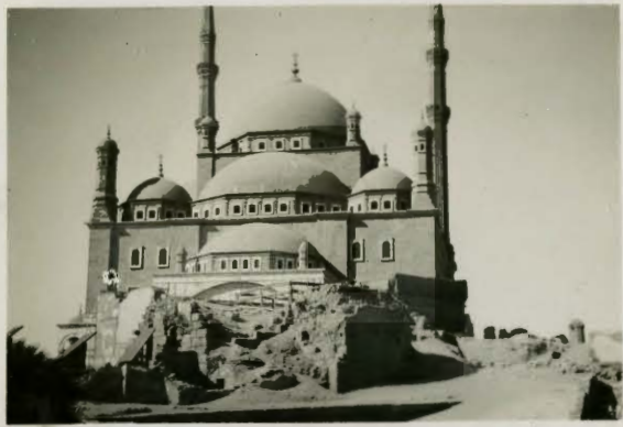
Dome & minarets of Alabaster Mosque
